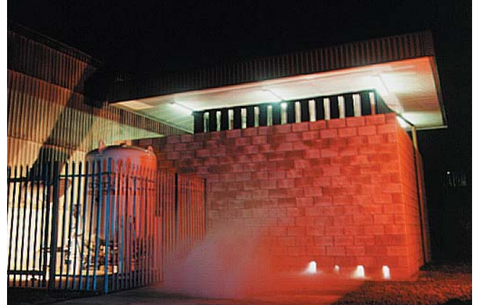
Cryogenic Test Facility/Explosion Proof Chamber.
